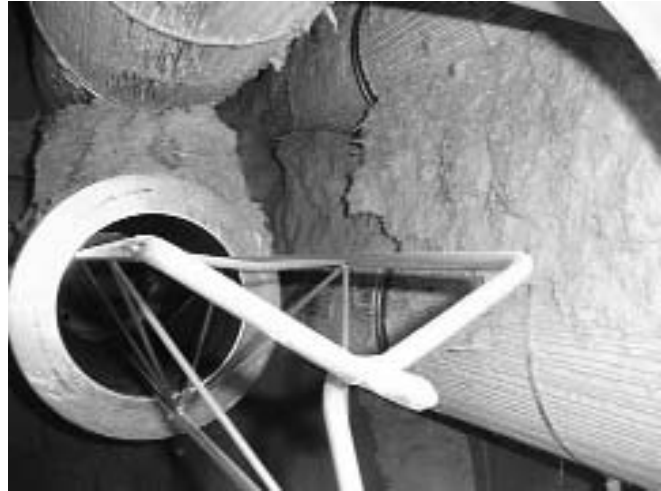
Figure 1 shows a top-loading problem in a horizontal filter system.
