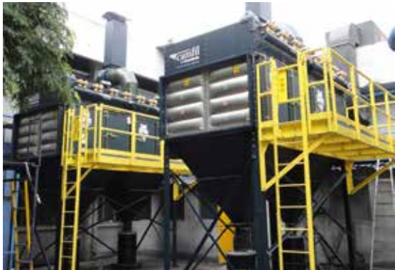
A pair of cartridge dust collectors with vertically-installed filters serve two metal spray booths for spraying zinc and aluminum in the manufacture of electronic components. The units successfully replaced previous dust collectors with horizontally-mounted filters that were performing poorly.
