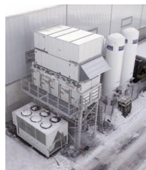
A view of the heat exchange system installed above the dust extractor.
