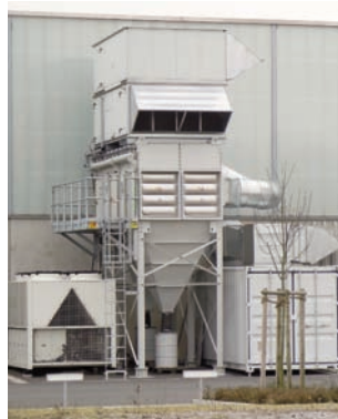
A Farr Gold Series® GS40 heat dust extractor located at Thermico's factory, in Dortmund, Germany.
