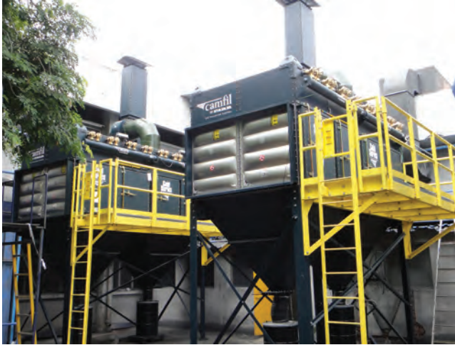
Both GS32 dust collectors are in place after replacing two horizontal filter-mount collectors at Vishay Components.
