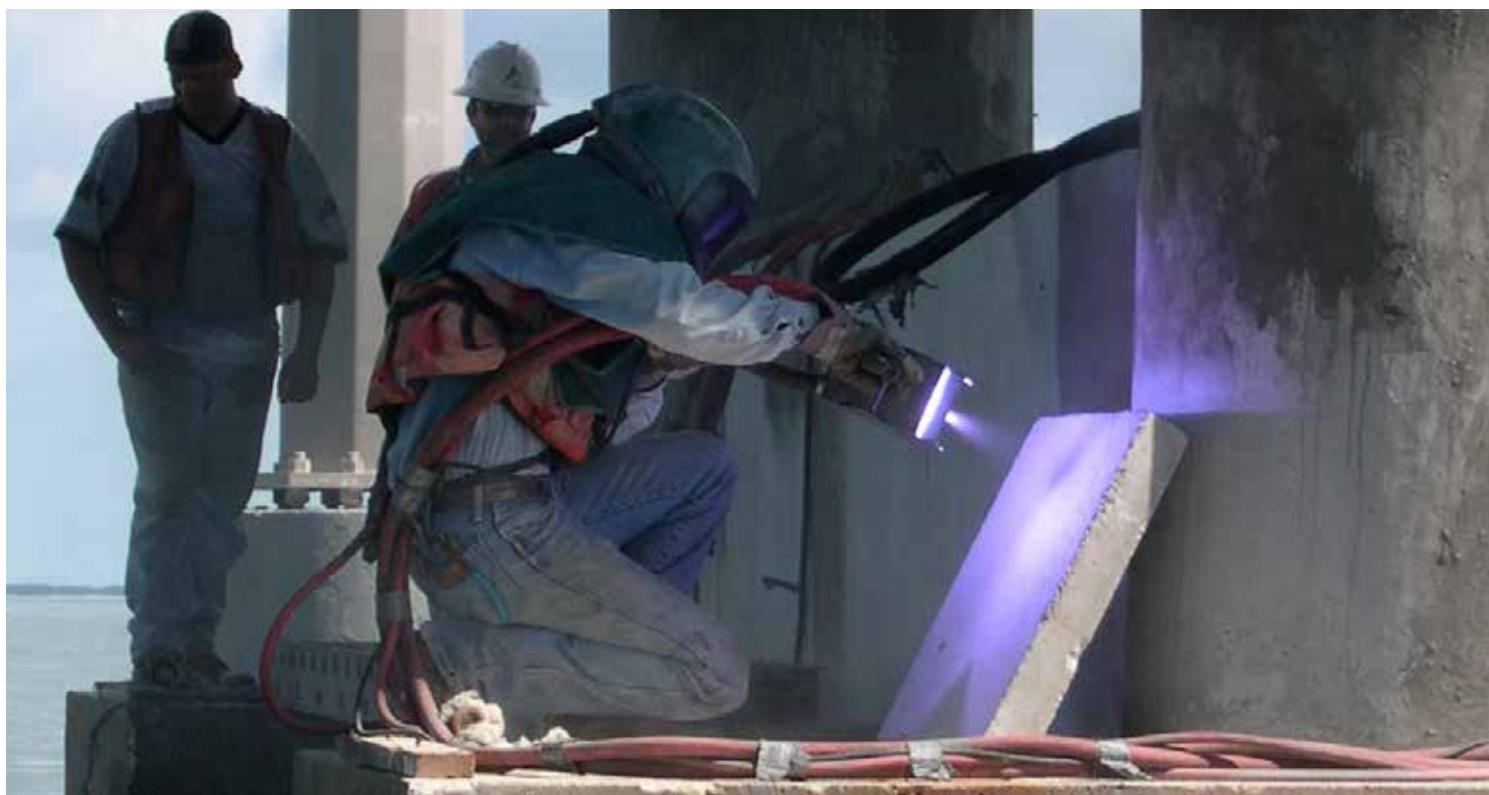
Fig. 4 — Preparation of a job reference standard prior to commencing production work.
