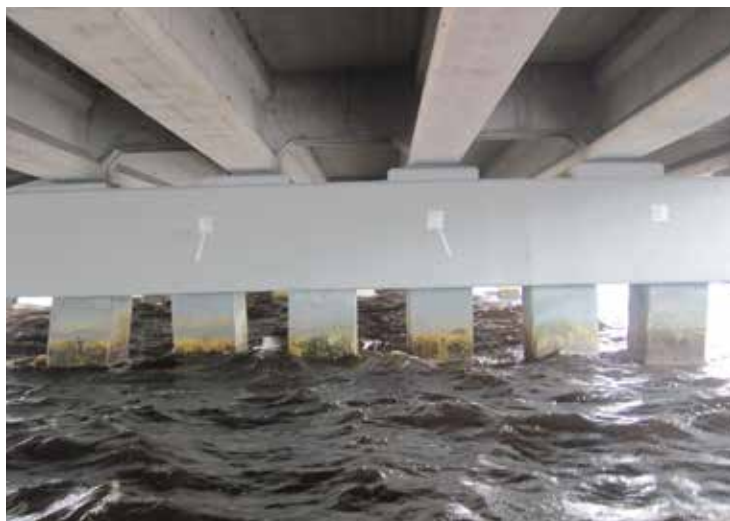
Fig. 3 — Application of sprayed zinc anode on concrete on a structure in a marine environment.
